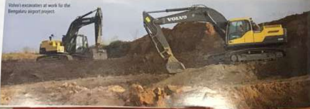
Volvo excavator at work for the Bengaluru airport project.
